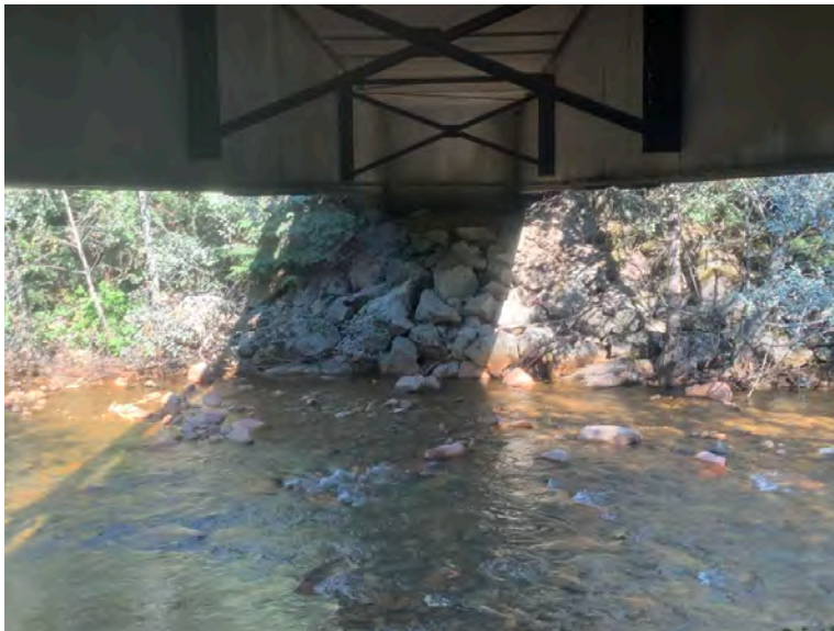
Left Bank Abutment when facing downstream
