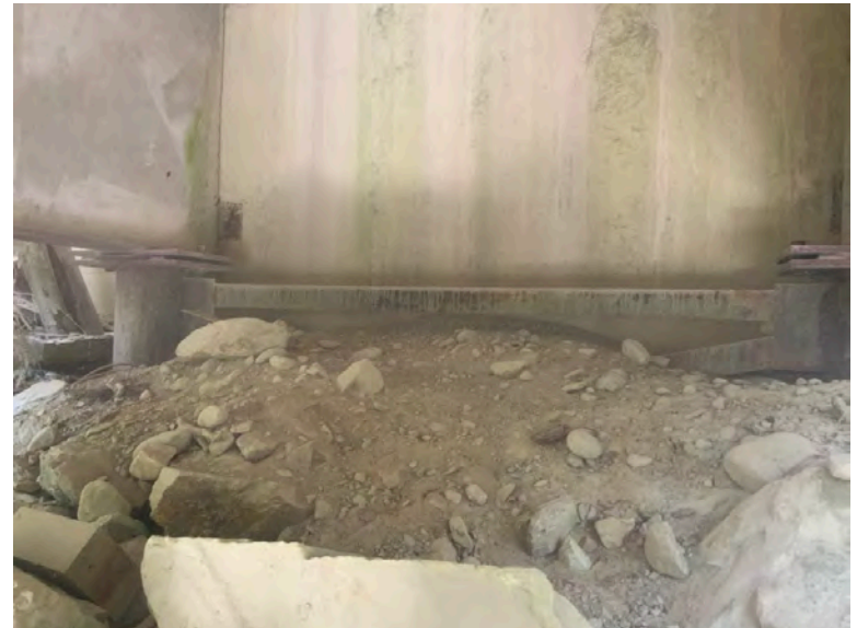
Left Bank Abutment when facing downstream
